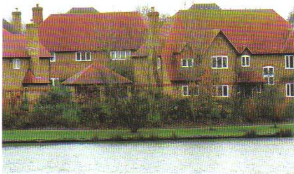
South East homes: infrastructure must accompany development
