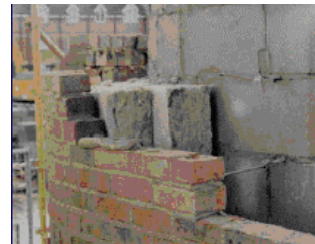
Super Insulation in situ.
