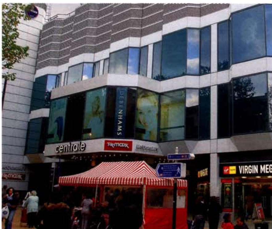
Croydon: commercial schemes earmarked to deliver integrated micro-renewable energy systems
